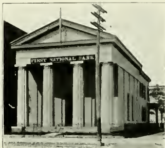
OLD FIRST NATIONAL BANK BUILDING.
